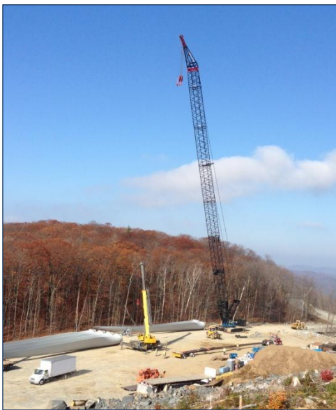
The 311 ft. tall Manitowoc 16000 crane is assembled on-site.
