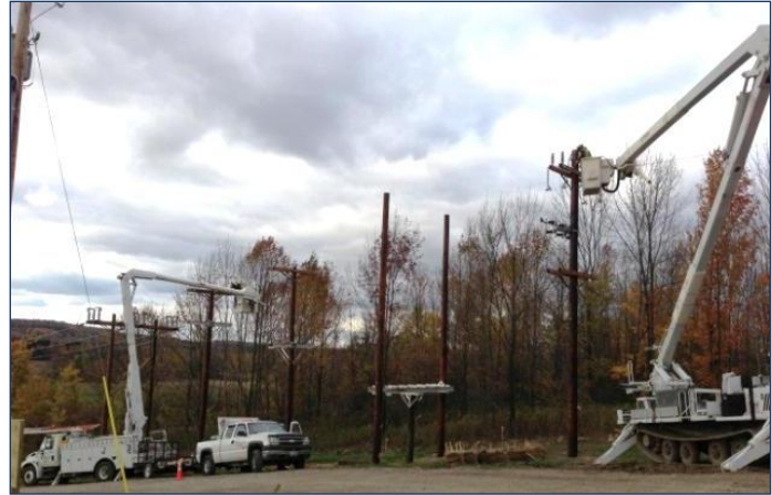
Workers continue construction on the overhead electrical system.
