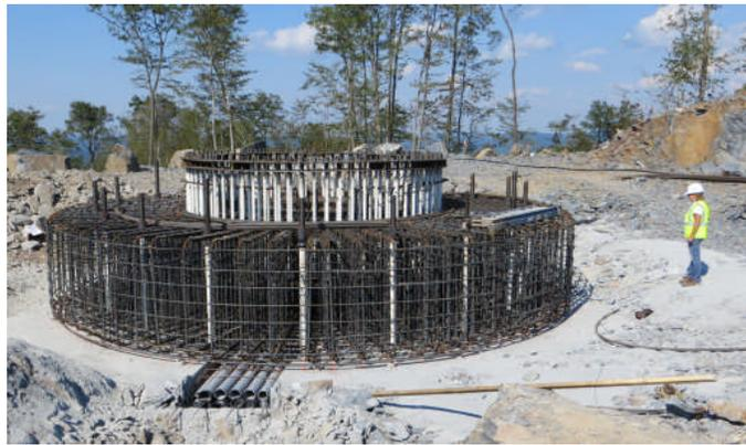
*Turbine foundations contain a large amount of steel 're-bar' as seen here in Turbine 3 before the concrete is formed and poured.*
