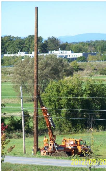
*GMP Crews set new poles along North Road to connect the project to the electric grid. (Credit RLC Eng)*
